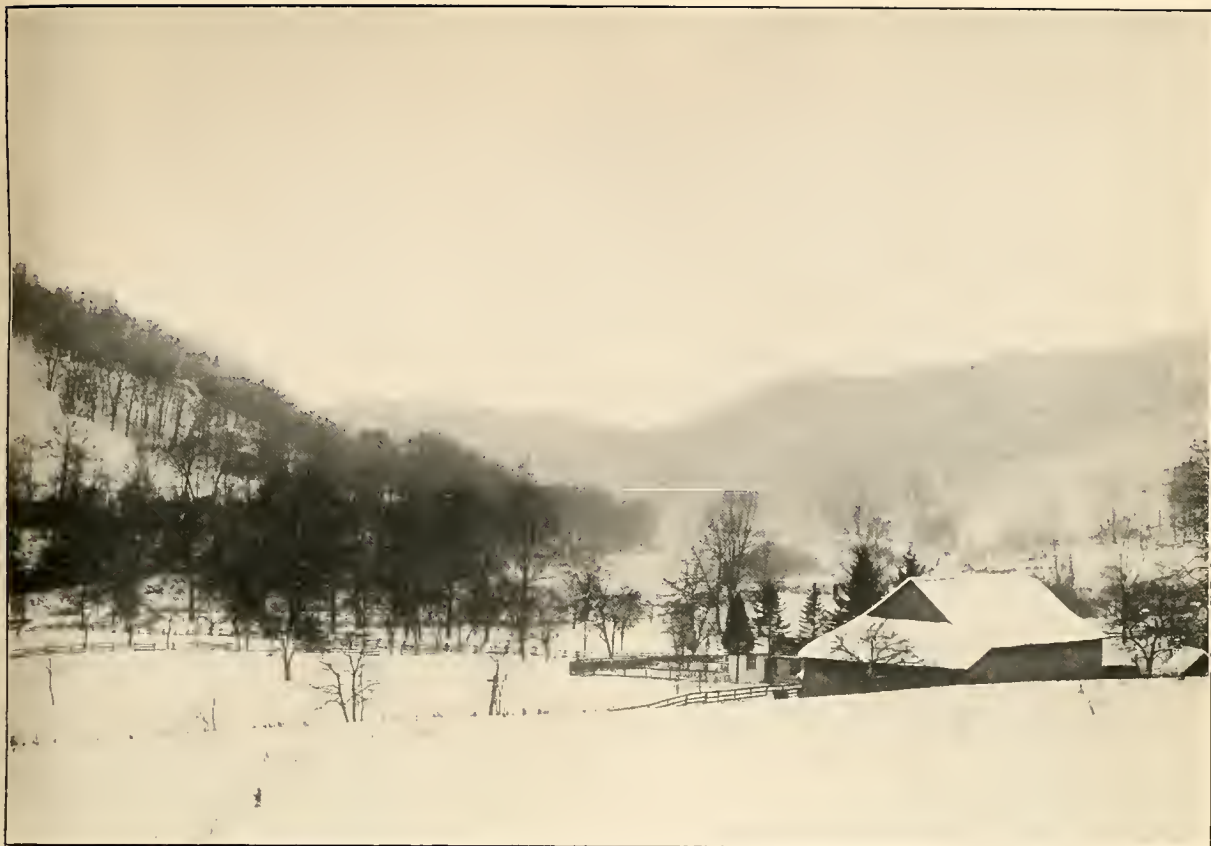
YOUGHIOGHENY RIVER, PA., DECEMBER, 1910. View up stream, showing crest of proposed Dam No. 1.
